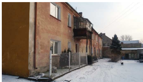
Photo 1. Building on the street 1 Maja 8.
